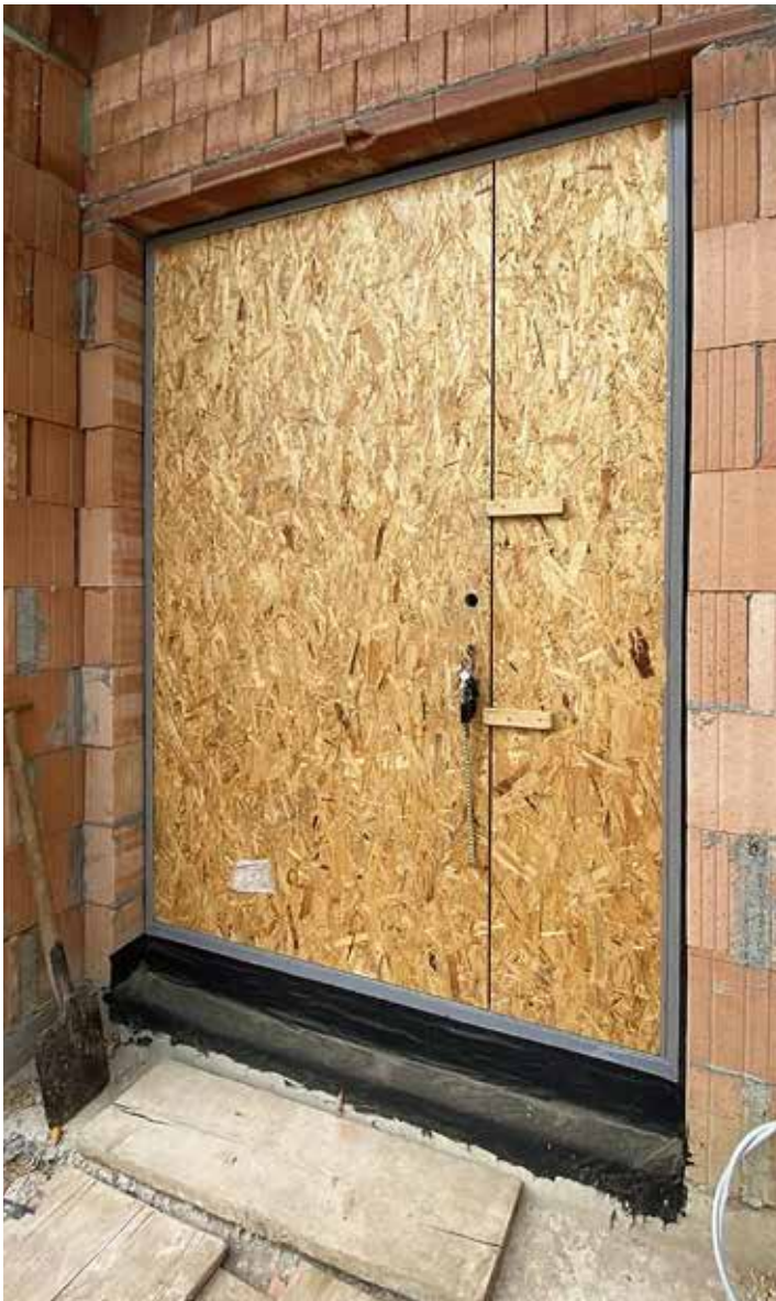
A temporary site door with a simple lock serves as a temporary closure at the entrance until the front door is installed. Finstral supplies temporary site doors ex works on request.
