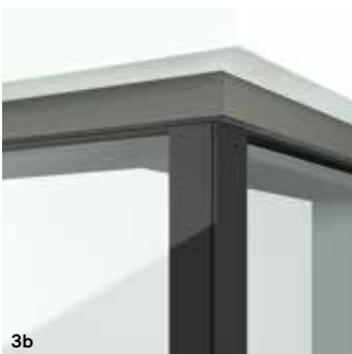
Corner coupling with all-glass corner, exterior
